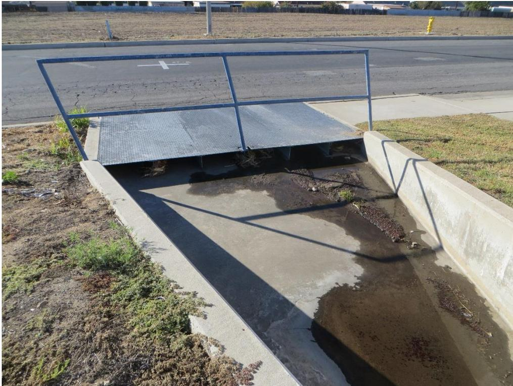
**Photograph 6:** The cement channel in Photograph 5 drains directly onto Bonnie View Drive, south of the project site. With project implementation, water would still flow onto the street via a culvert under a new pedestrian walkway.
