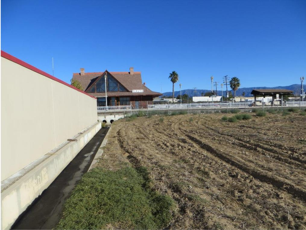
**Photograph 5:** A non-jurisdictional cement channel runs immediately west of the project site. It drains water underneath the railroad tracks. This channel would be covered with a pedestrian walkway to the Metrolink station in the distance but water would still run underneath.
